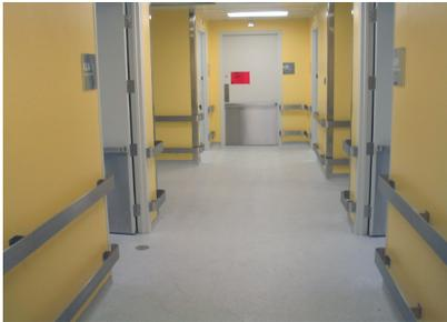
Various Tnemec coatings, including Series 273 Stranlok ML, a fiberglass mat-reinforced epoxy, were specified for the floors, walls & ceilings of the critical research areas at the University of Toronto Terrence Donnelly Centre for Cellular & Biomolecular Research.
